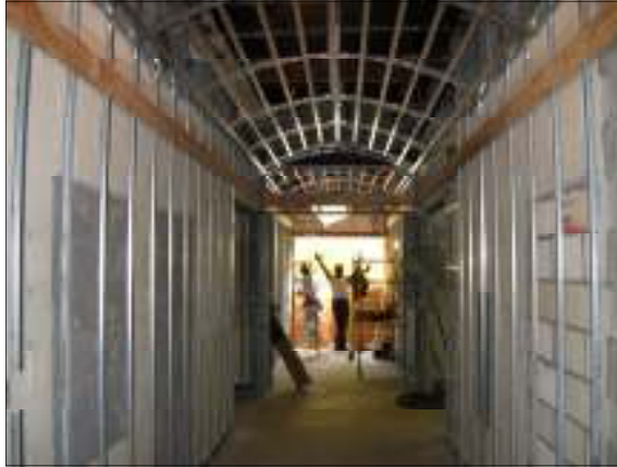
Looking from new Fellowship Hall—kitchen on left.
