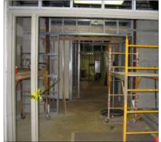
Looking from Contemporary Service space.
